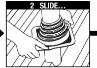
Slide Master Flash down over pipe (A non-petroleum base lubricant will ease installation).
